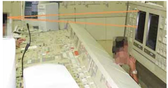
Fig. (5). From his position the operator cannot see the entire display.
