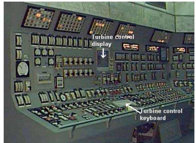
**Fig. (1).** Turbine display and keyboard together with analog instrumentation.
